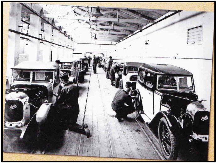
The Swallow Sidecar Company's assembly line at Coventry assembling Austin Seven Swallows.
